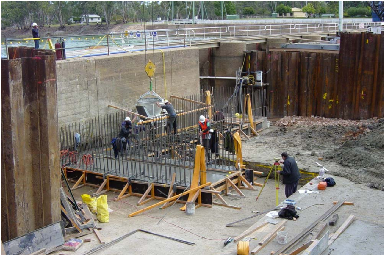
Construction of New Fishway at Lock 8 (Wangumma)
